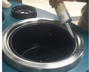
7. Allow the sealant to cure per the sealant manufacturer's instruction before using the drop-in.
